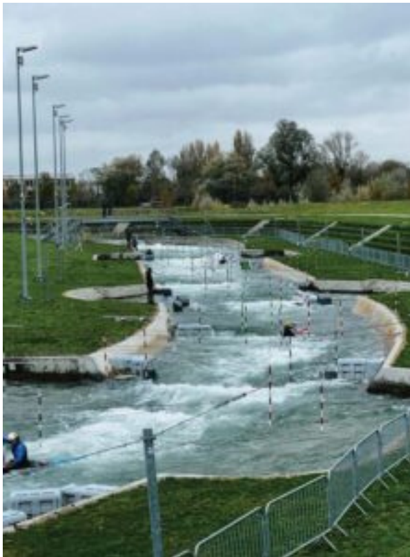
The kayaking facility for the Paris 2024 Olympic Games
